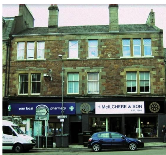
Fig. 3. The Bakery, 19 Main St, Campbeltown
